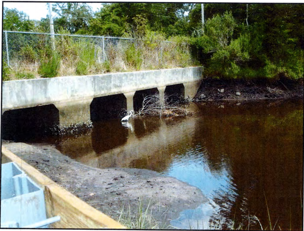
Exhibit 1. Box Culvert Under San Pablo Road (1/18/2008)
